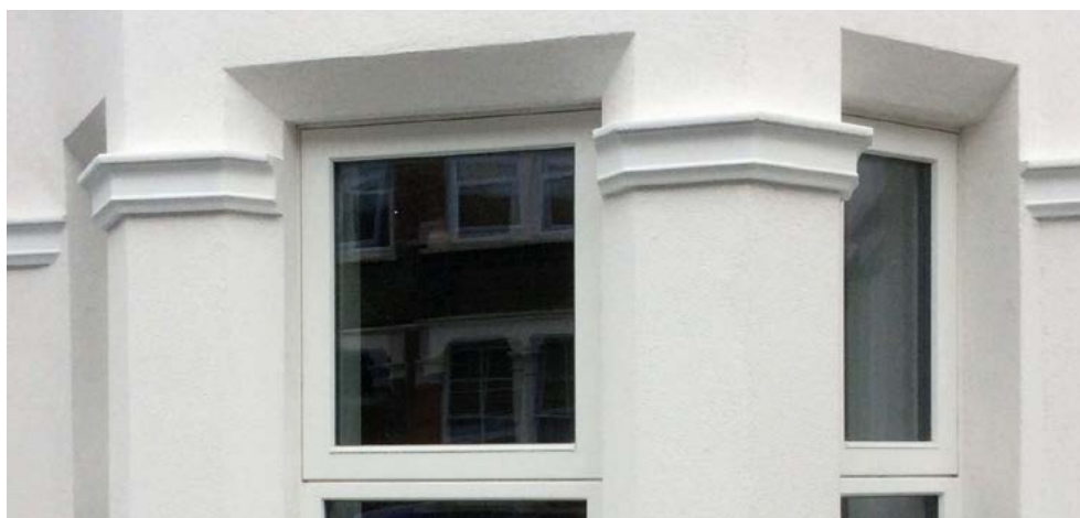
Figure 6 Example of externally splayed reveals
