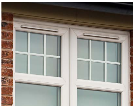
Figure 8 Trickle vents incorporated in a casement window
