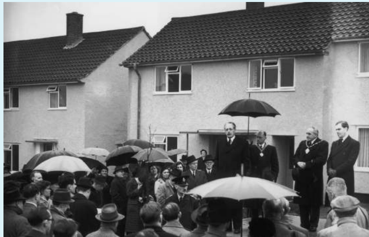
Harold Macmillan, Minister of Housing and Local Government, opens Eastcote Estate houses in Middlesex, 1952. The houses, built by Wimpey, were erected in seven weeks.
