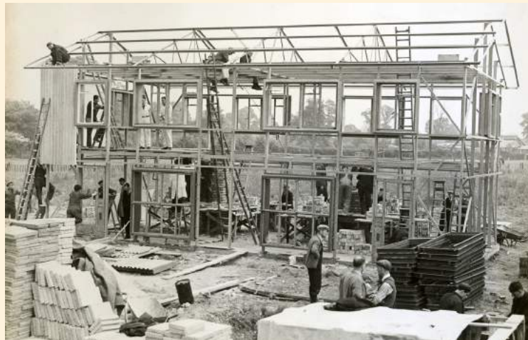
British Iron and Steel Federation (BISF) prefabricated house at the Ministry of Works' testing ground, Northolt, London, 1939–1945
