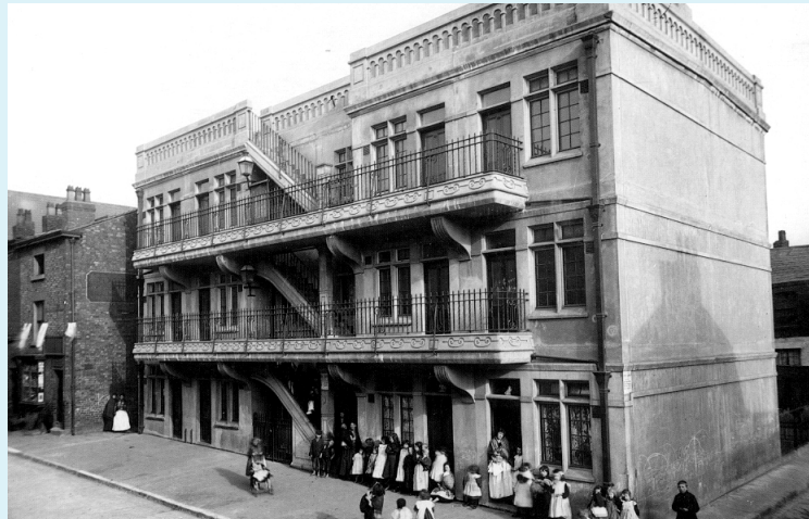
Eldon Street Labourers' Concrete Dwellings, Liverpool, 1903–1905
