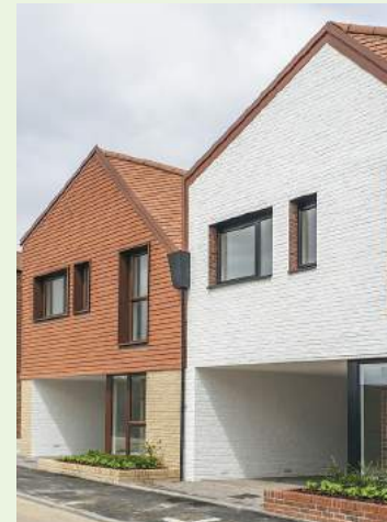
Swan’s Beechwood West, Basildon, 2019, first phase includes 30 modular homes
