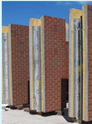
Insulated panels provide a ready-made external envelope with various finishes
