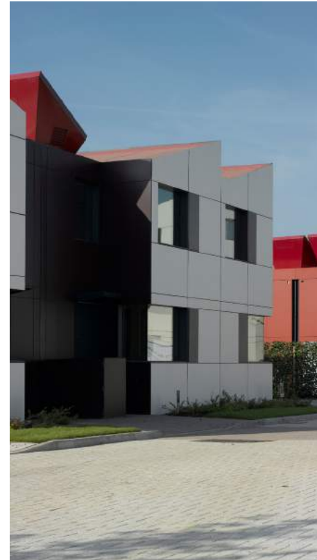
Oxley Woods prefabricated timber frame sustainable housing development, Milton Keynes, 2007
