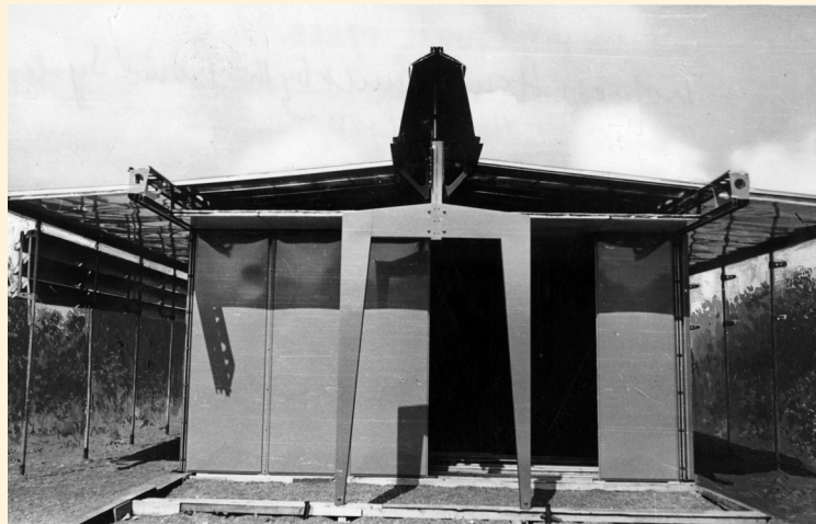
Maison Tropicale by Jean Prouvé under construction, 1951
