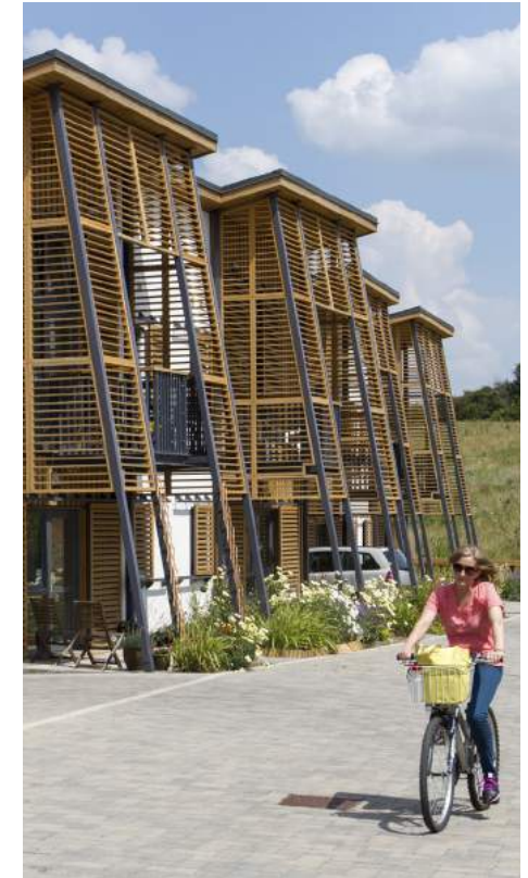
Hanham Hall eco village structural insulated panel system (SIPS) construction, Bristol, 2015
