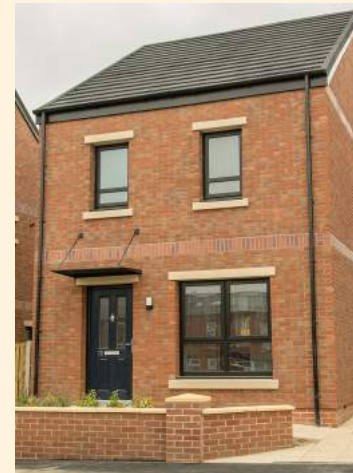
St Hilda's, Leeds, 2018: built using a light steel frame panellised system
