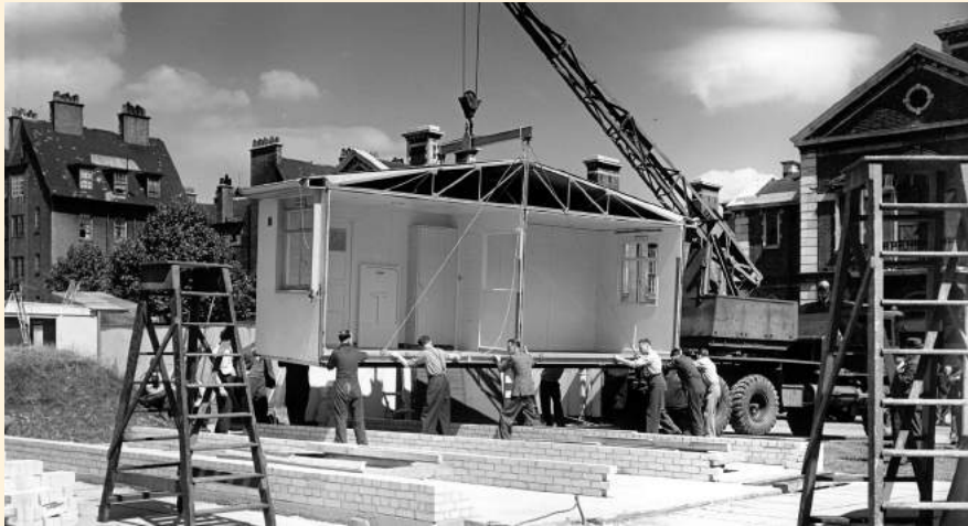
AIROH prototype house under construction, Tate Gallery, London, 1945
