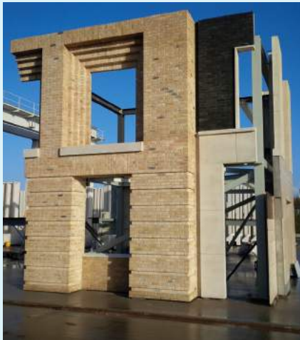
Garden Halls, Kings Cross, London, 2017, by TP Bennett/Maccreanor Lavington providing 1,200 student rooms and constructed from around 1,100 precast panels incorporating 4 brick types
