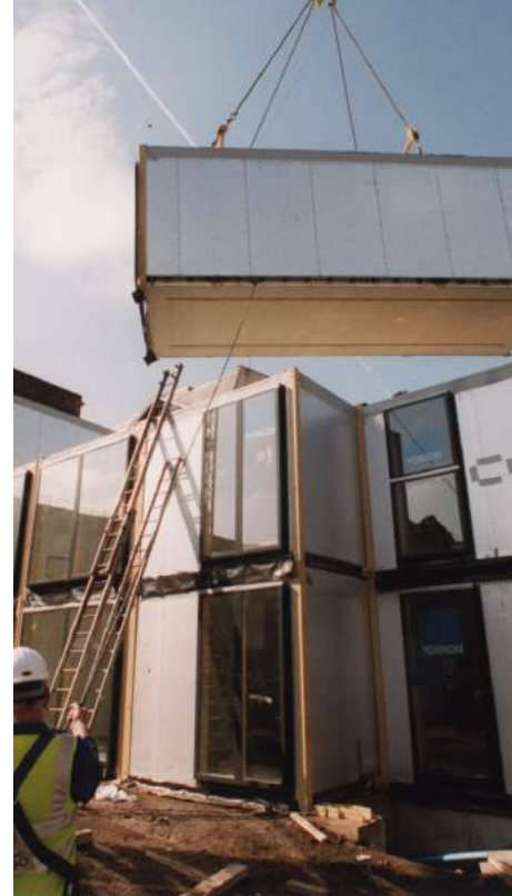
Murray Grove, London, 1999, volumetric construction using light steel frame for dense urban housing
