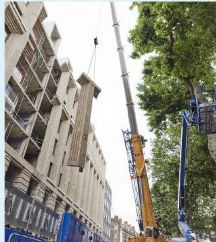
Garden Halls, Kings Cross, London, 2017, by TP Bennett/Maccreanor Lavington providing 1,200 student rooms and constructed from around 1,100 precast panels incorporating 4 brick types
