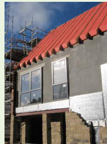
Timber cassette roof at Derwenthorpe sustainable community, York, 2013
