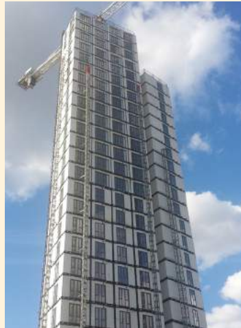
Mapleton Crescent: factory-made modules delivered, stacked and linked
