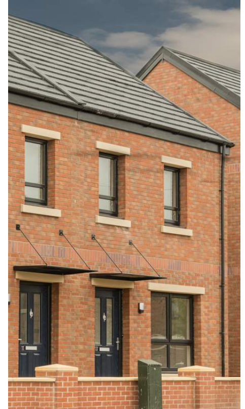
St Hilda's, Leeds, 2018, panellised construction using light steel frame for low-rise family homes
