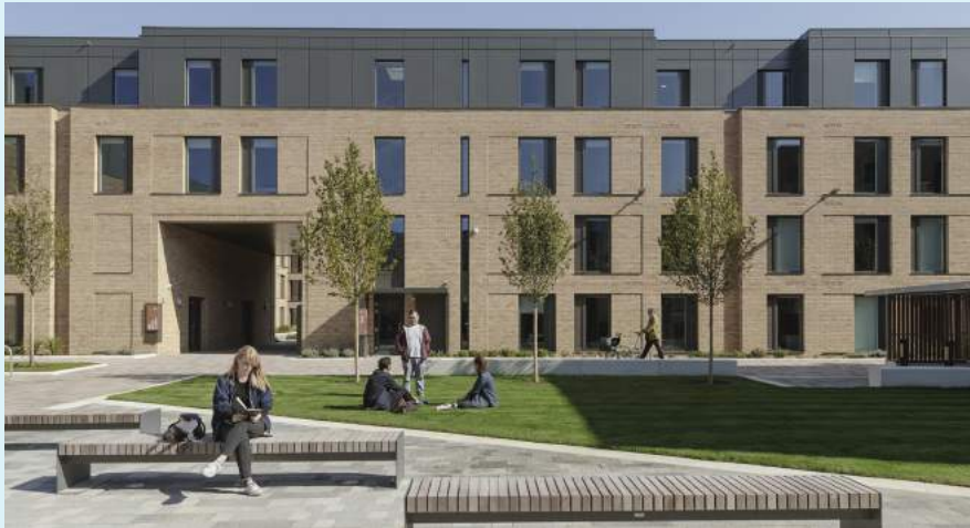
Hox Park, Egham, Surrey, 2018 by Studio Partington provides 500 student rooms using a prefabricated concrete superstructure, bringing cost, programme, resilience and environment benefits
