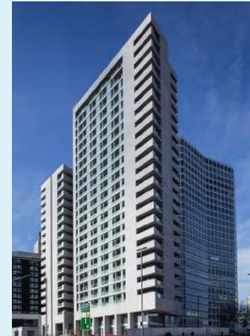
Arena Central, Birmingham, 2019 using up-to-date precast construction
