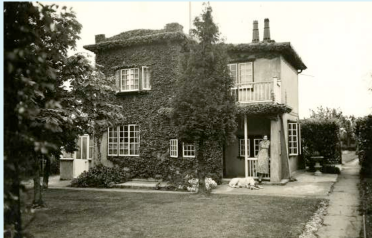
158 Wilbury Road, Letchworth, 1905, Grade II* listed both for its style and its radical prefabricated reinforced concrete construction
