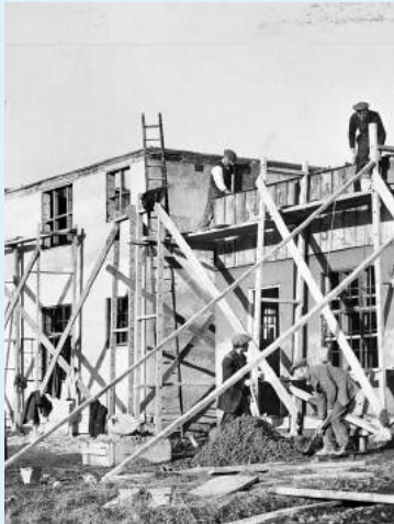
Easiform cast-in-situ concrete housing being constructed in 1926
