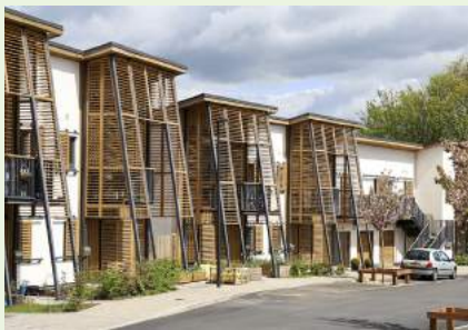
Hanham Hall deep roof overhangs, balconies and shutters help avoid overheating in summer
