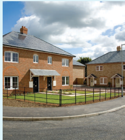
Brookwood Farm, Woking, 2009: ICF construction with traditional appearance
