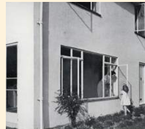
Letchworth Cottage No. 47 by New Expanded Metal Co. Ltd, 1905. Innovative use of metal lathing as a base for external render and internal plaster finish
