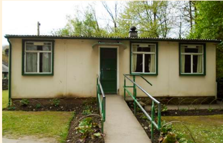
AIROH prefab, St Fagan's Museum, Cardiff: a forerunner of 'volumetric' construction
