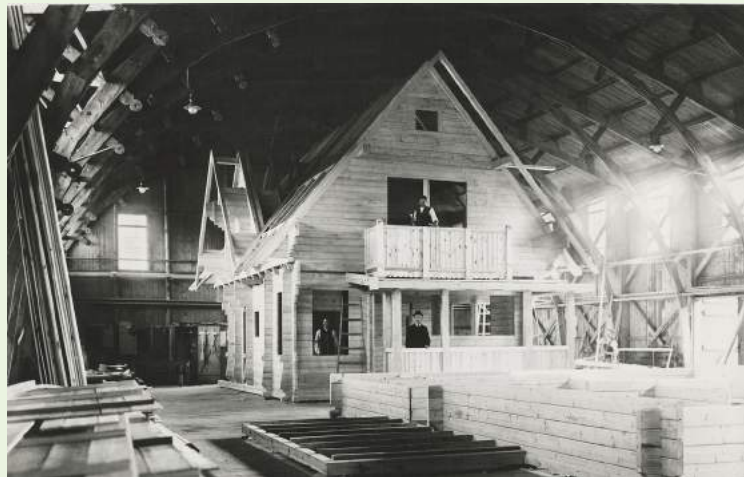
Christoph & Unmack Assembly Hall, Niesky, Saxony, Germany. Houses were assembled and disassembled before they were sent to their destinations
