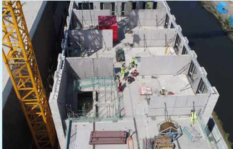
Example of precast concrete cross wall construction, a fast and convenient way to produce multi-unit structures
