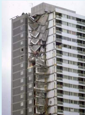
Ronan Point infamously collapsed in 1968 denting confidence in prefab high-rises
