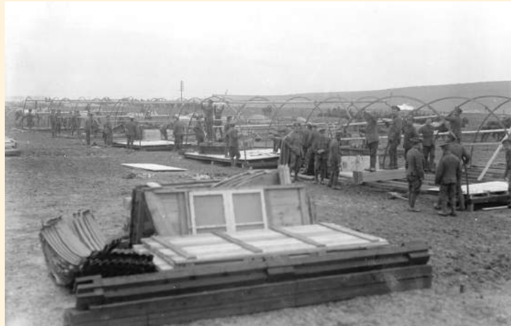
British troops constructing Nissen huts, Fricourt, 1916
