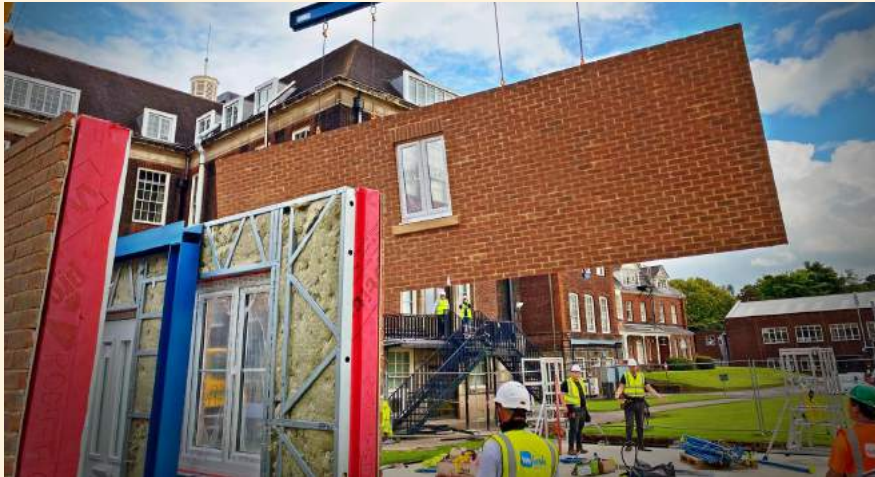
Light gauge steel frame open panels, lining materials installed on site
