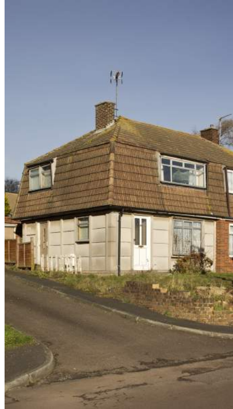
Cornish Unit precast houses at Hoo Peninsula, Medway, Kent. Thirty thousand built 1946–1960s
