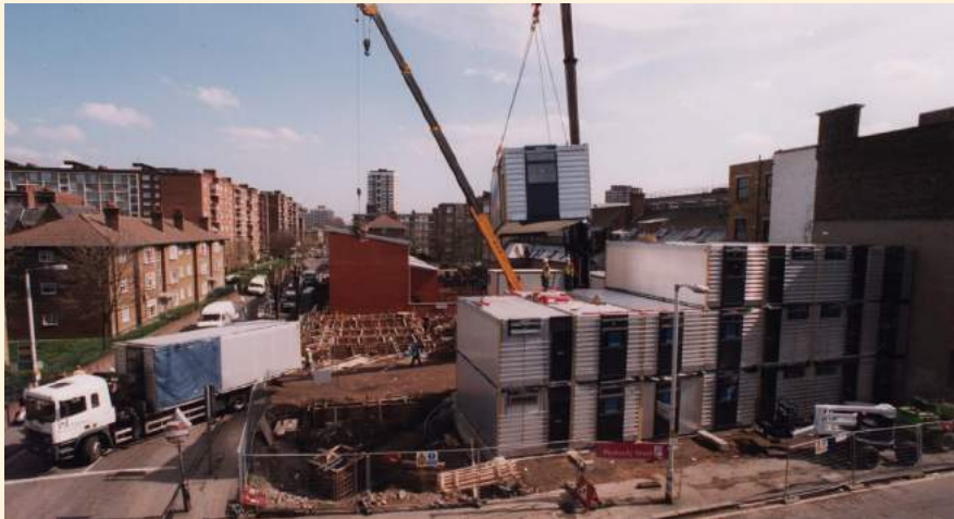
Murray Grove: the project was on site for just six months
