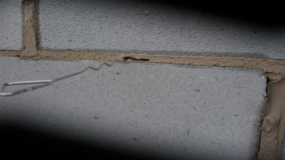
Tell-tale slot confirms ties installed after laying.
