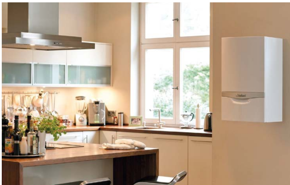
Figure 8 The indoor unit of a ground-source heat pump
