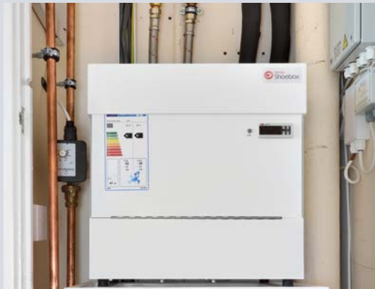
Figure 12 A shoebox-type heat pump in situ
