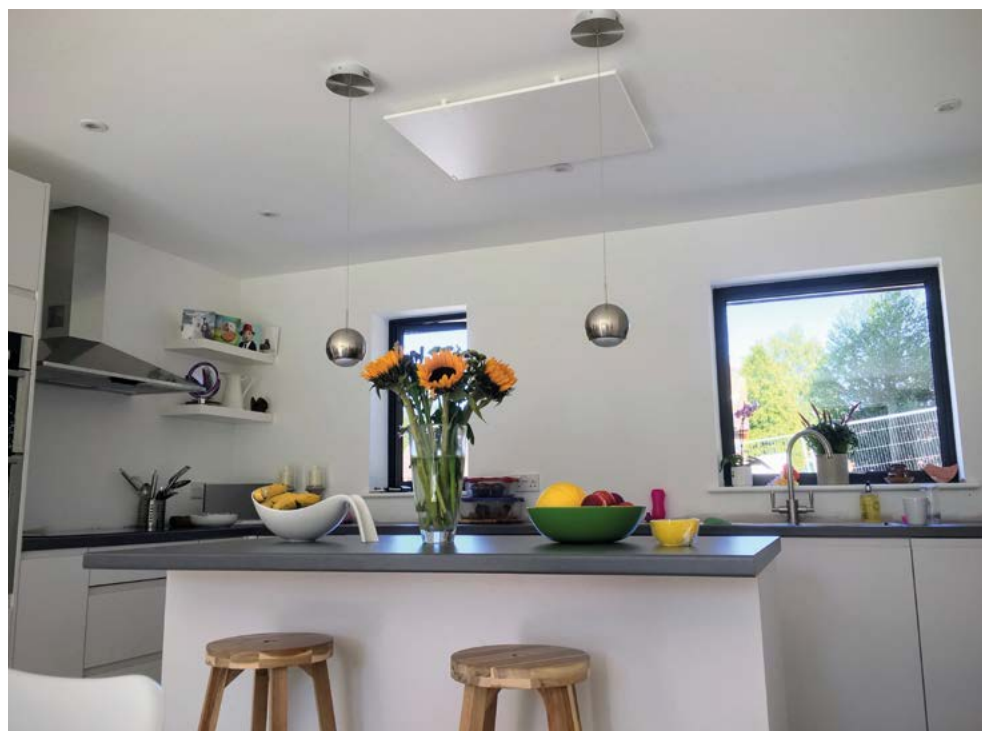
Figure 15 An infrared heating panel
