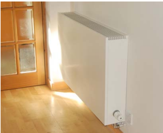
Figure 13 A low-temperature radiator
