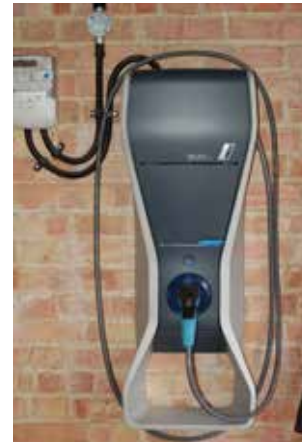
Figure 4 Typical residential chargepoint installations
